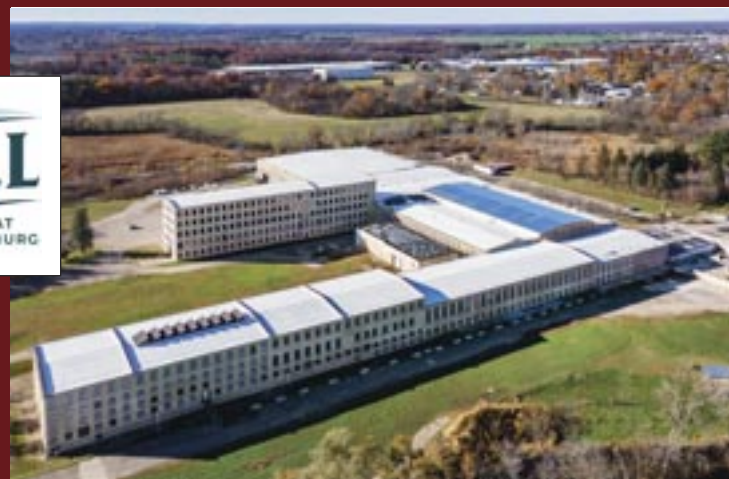
Before it became "The Mill at Vicksburg," this colossal, 420,000 square foot complex was the historic Lee Paper Company Mill, which sits on a 120-acre campus. This aerial photo was taken in November 2024 and shows the recently-completed new roof on the massive structure.
