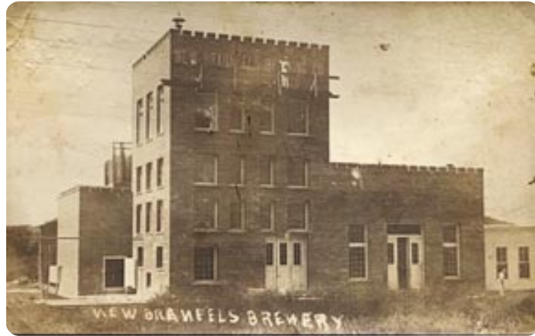
Real photo postcard showing worker on scaffold making repairs after the plane crash, c. 1921. Collection of John Rightmire.
