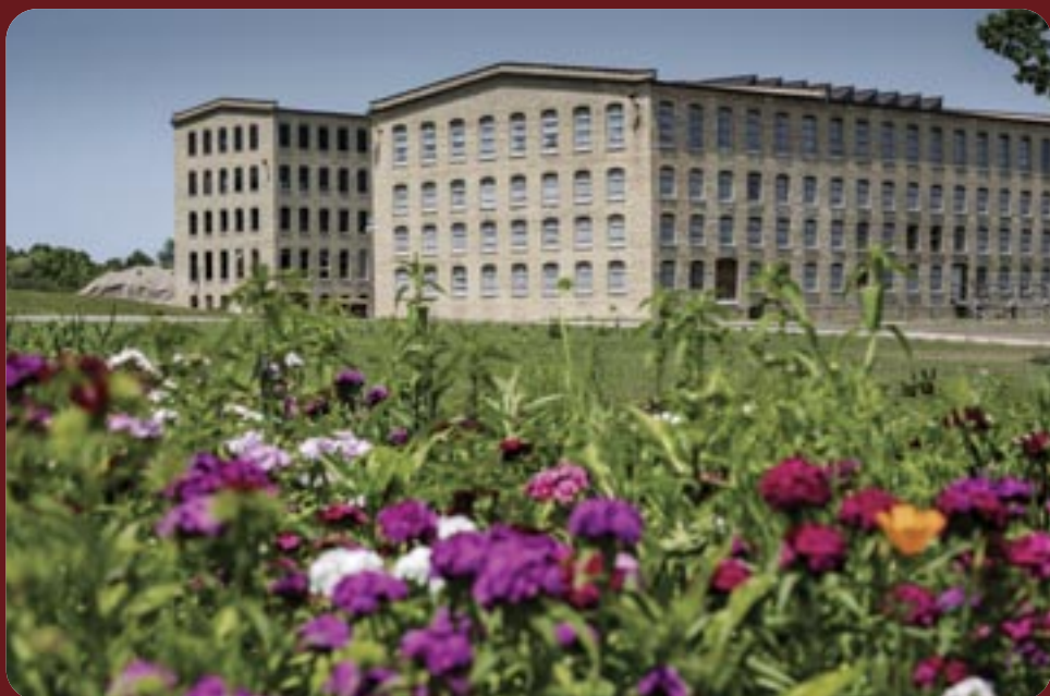
The expansive outdoor part of The Mill's campus will feature walking paths and nature trails highlighted by the property's large wildflower installation and water features.
